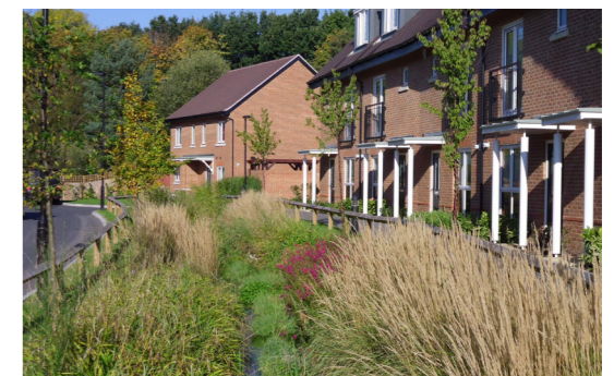
Vegetated swale integrated peri-urban streetscape
