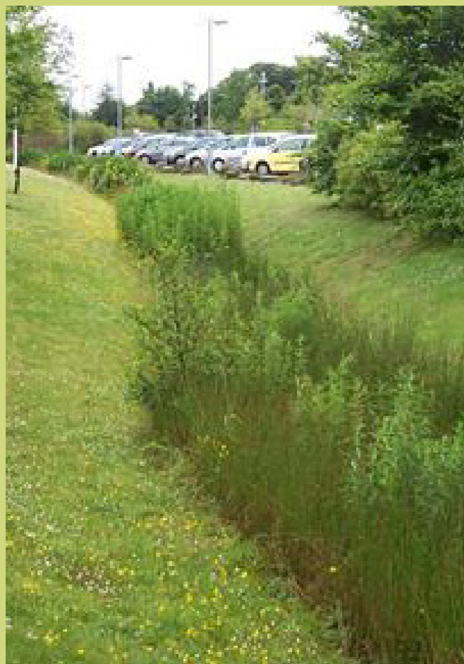
4. An example SuDS feature; swale
