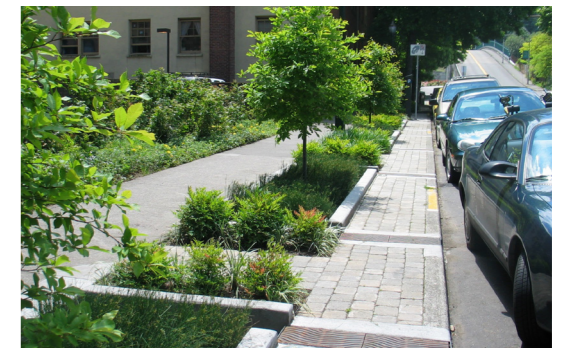
Urban canalised swales
