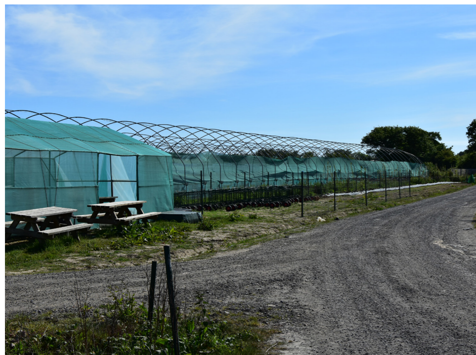
Photo 9. Polytunnels in the north of the Site Allocation
