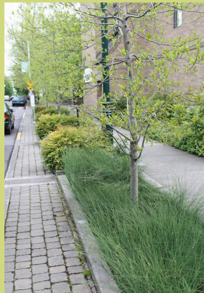
5. An example SuDS feature; roadside swale
