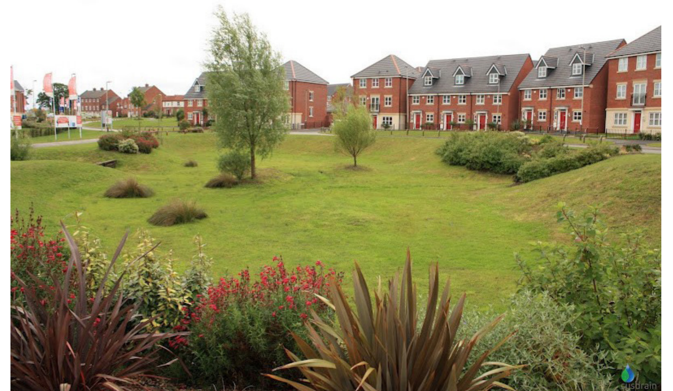
3. An example SuDS feature; Attenuation Basin (in dry conditions)
