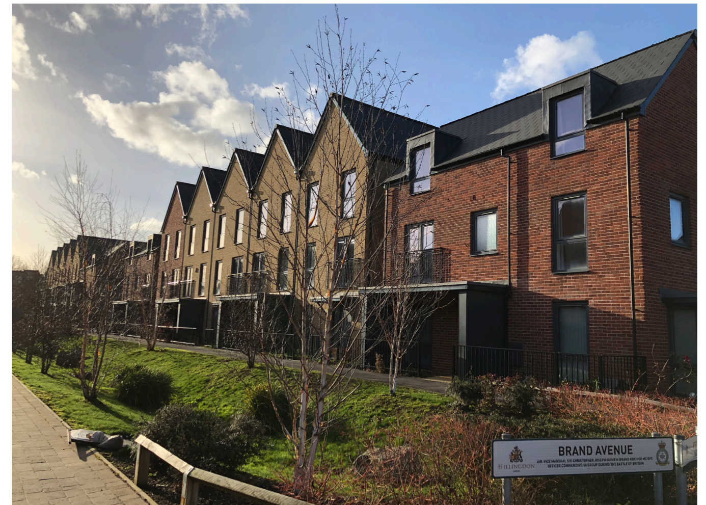
2. An example SuDS feature; a roadside swale, depth varies depending on requirements.
