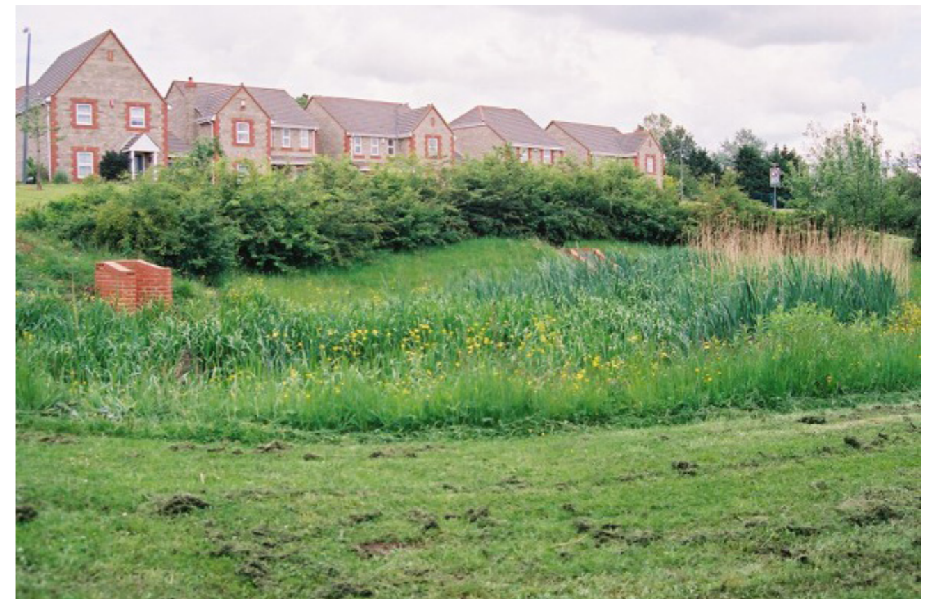
7. An example SuDS feature; a wetland area also providing large scale biodiversity benefits
