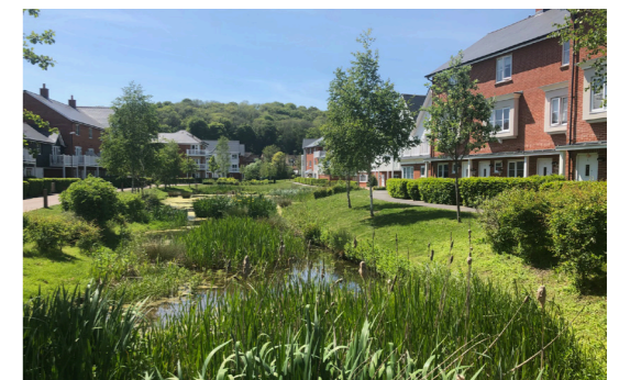
Vegetated swale integrated into semi-rural streetscape
