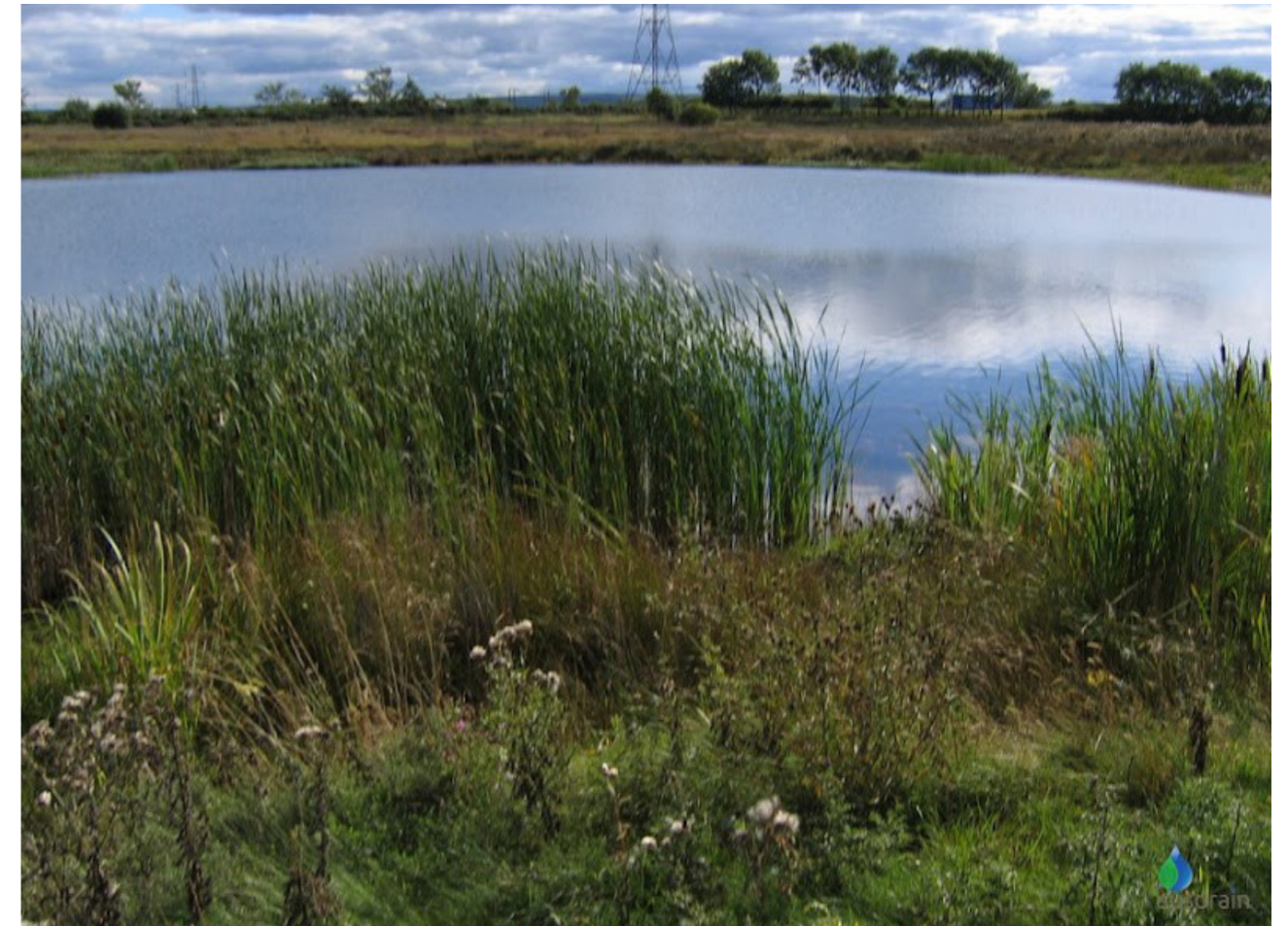
6. An example SuDS feature; attenuation Pond (in wet conditions)
