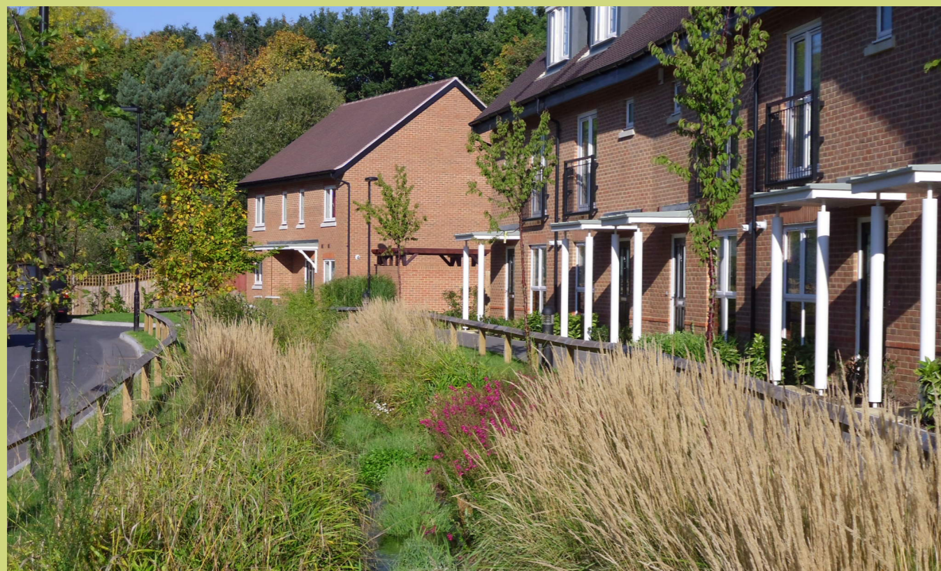
1. An example SuDS feature; a roadside swale, depth varies depending on requirements.
